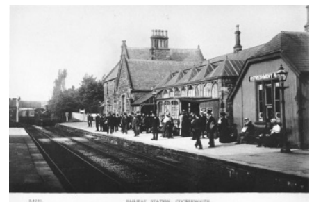
Cockermouth Railway Station
